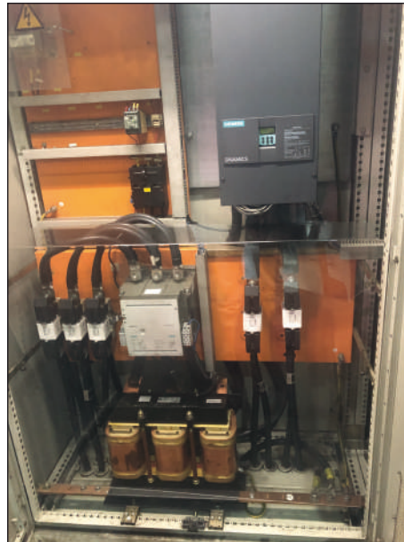
Obsolete frequency shifter cabinet
